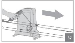
**06** • Open the gate to support the point of the new piece of rack on top of the pinion and weld the spacer.
